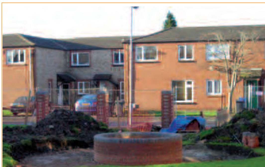
Bentley Road under construction
