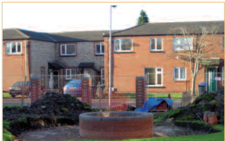
Bentley Road under construction
